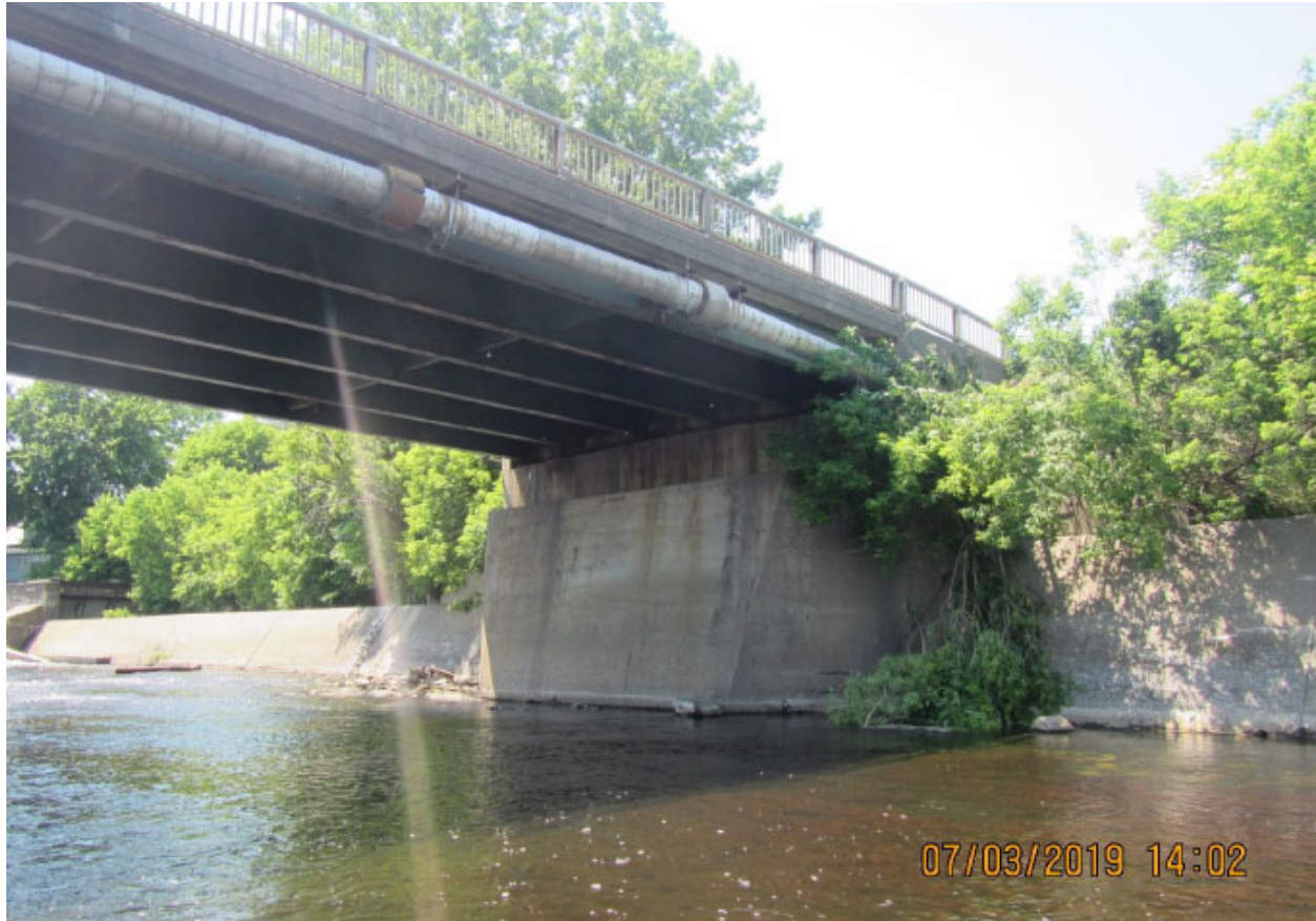
Figure 5. Facing northern abutment. Note utility on bridge and retaining walls adjacent to abutment.
