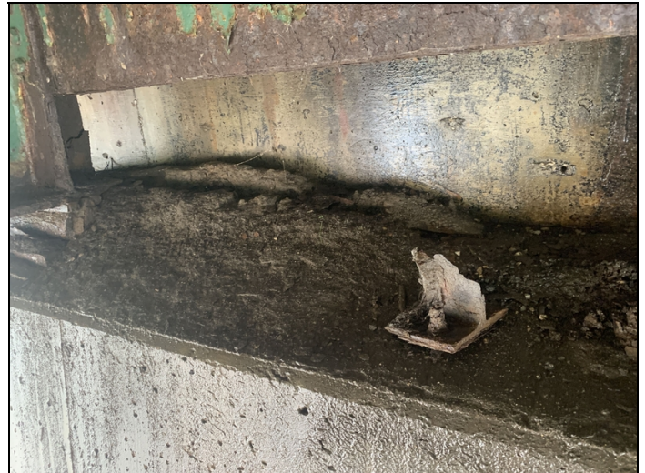
abutment 1 seat area
