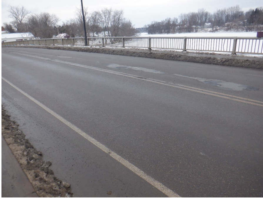
Photo 1: Bridge 6 – Typical Top of Deck, Looking Southeast
