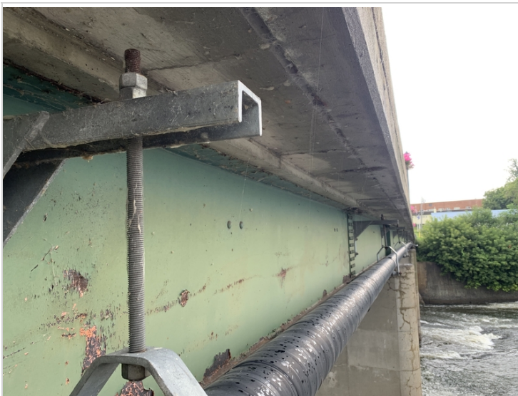
Beam 6 looking east
