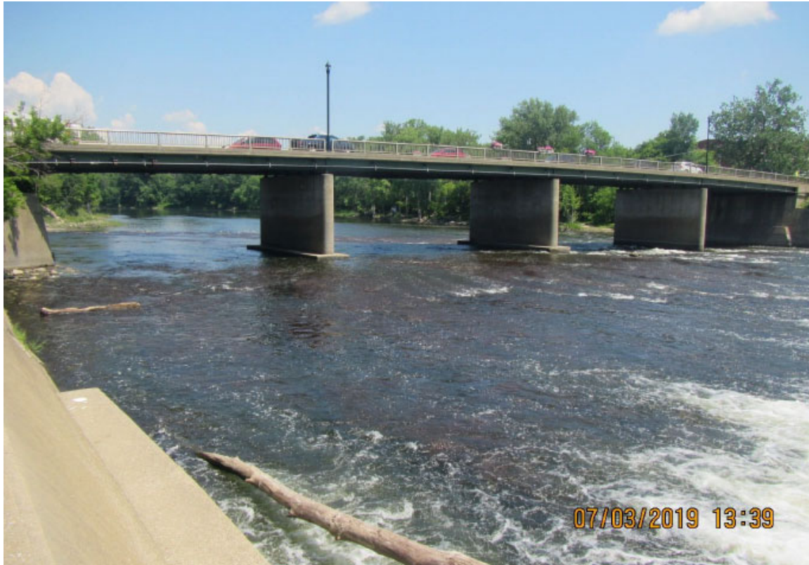
Figure 3. Facing upstream at structure, note pier locations and utilities
