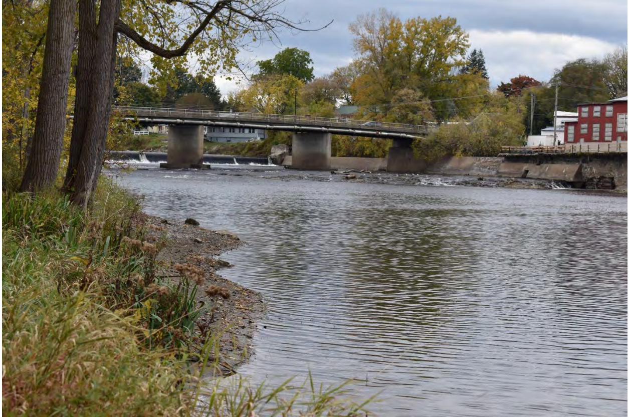
Figure 22. View west of bridge BR 6 from the southeast quadrant of the proposed Swanton BF 036-1(16) Project in Swanton, Franklin County, Vermont. The photo was taken from the river bank immediately north of ASA 3.
