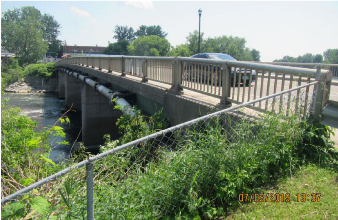
Figure 1. Facing south at northern end of bridge. Note utility alongside bridge for full length, and light pole on bridge.
