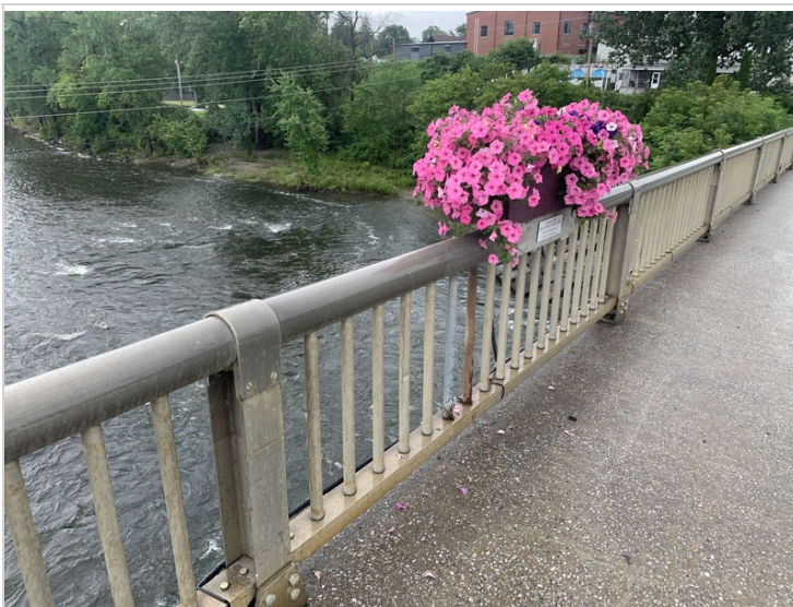
Downstream near pier 1 rail spindles
