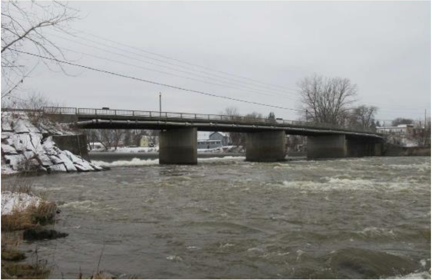
Bridge No. 6, Swanton. Image from WSP report.
