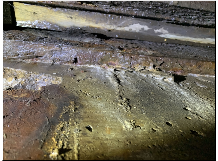
Wood used to support joint abutment 1
