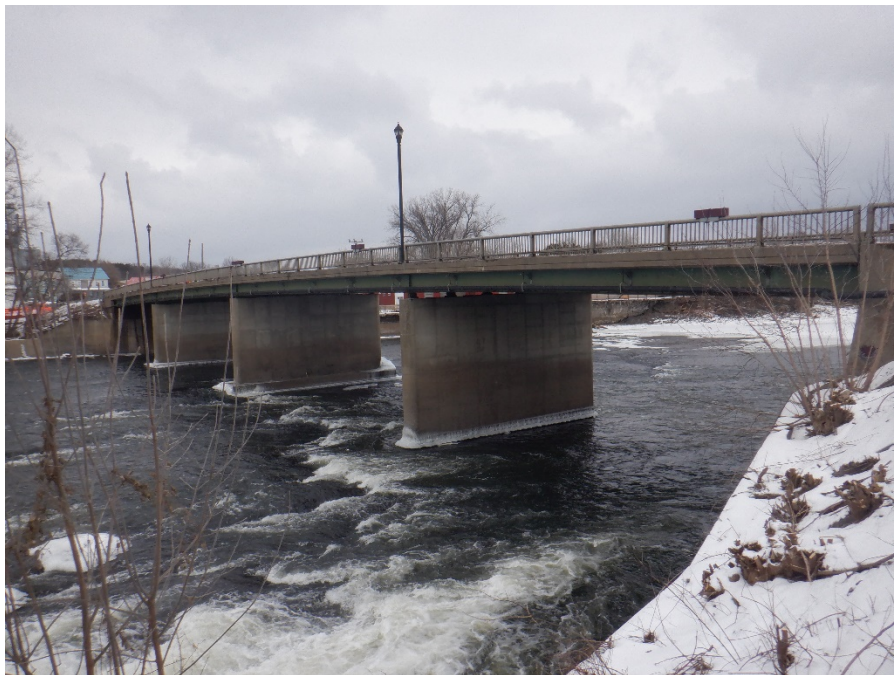
Photo 6: Bridge 6 – South Elevation, Looking North
