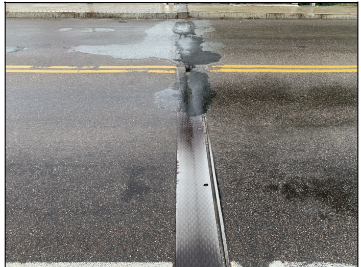
Abutment 1 joint
