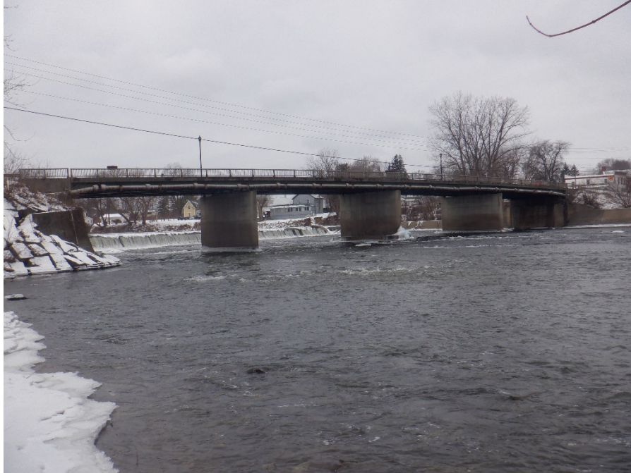
Photo 7: Bridge 6 – North Elevation, Looking South
