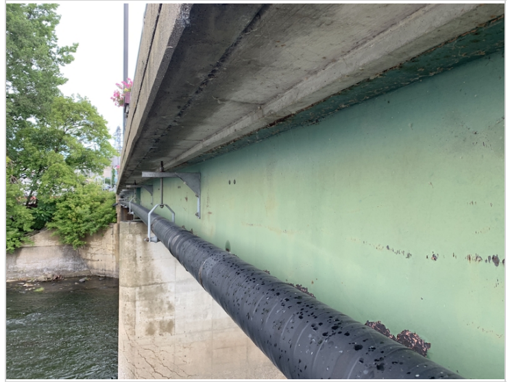
Beam 6 looking west
