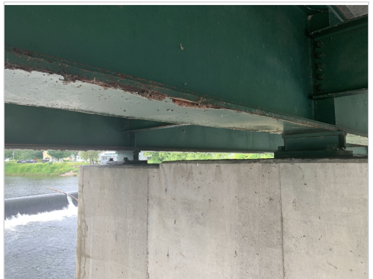
Pier 2 fixed bearings beams 5,6
