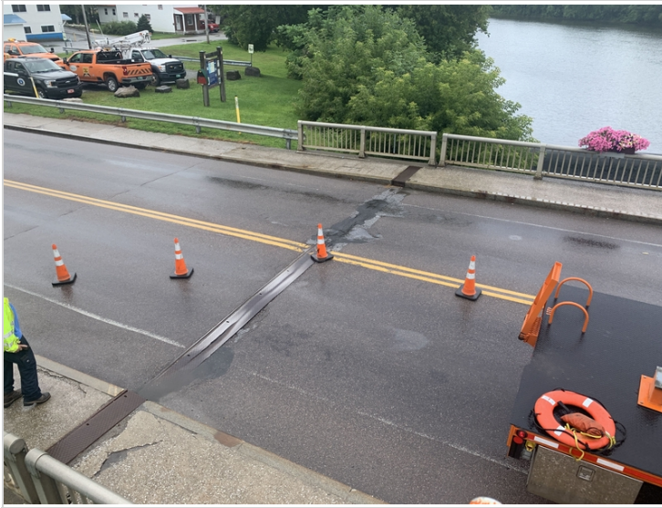
joint abutment 1 patching
