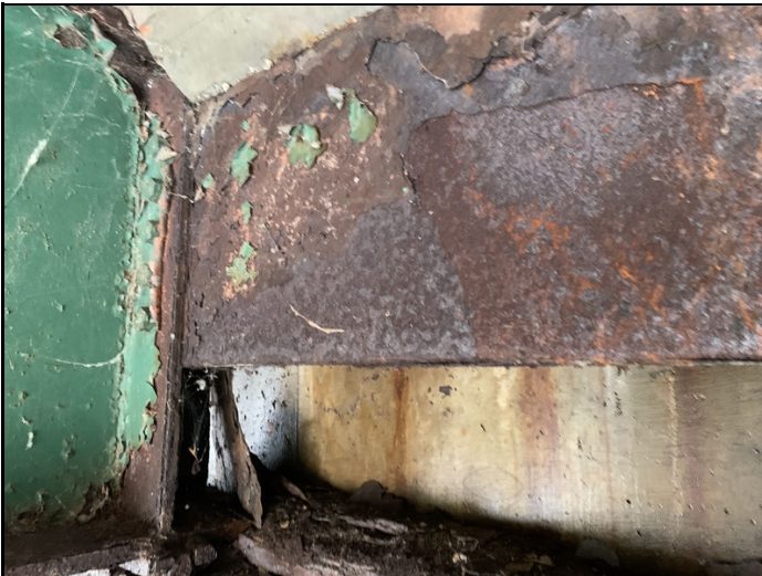
End diaphragm's abutment 1
