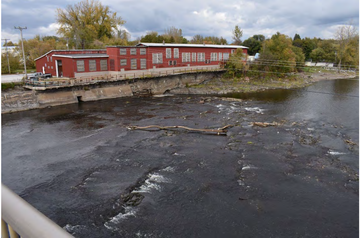
Figure 24. View northeast of the northeast quadrant of the proposed Swanton BF 036-1(16) Project in Swanton, Franklin County, Vermont, showing the former Vermont Marble Company marble cutting mill building. The photo was taken from the Route 78 bridge, the guardrail of which is visible in the lower left corner.
