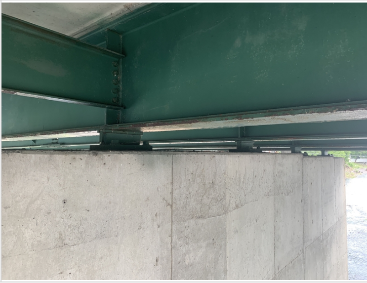
Pier 2 fixed bearings beams 1-4
