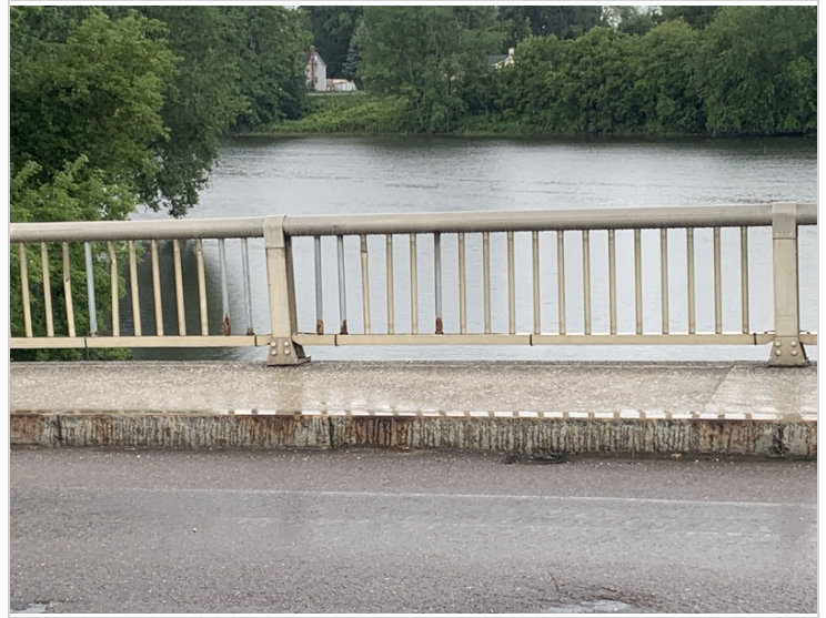
Upstream near abutment 2 rail spindles
