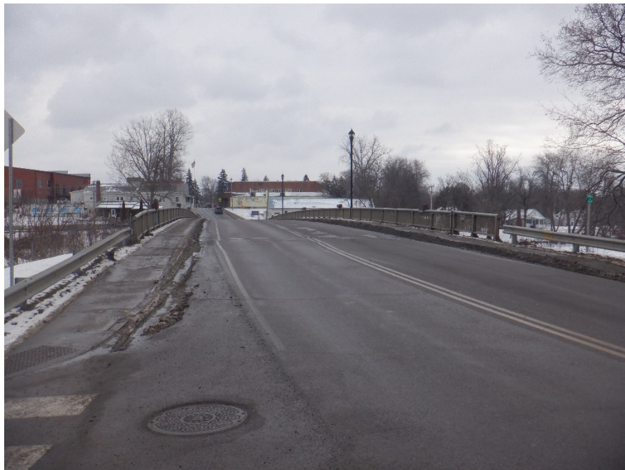
Photo 2: Bridge 6 – Bridge from West Approach, Looking East
