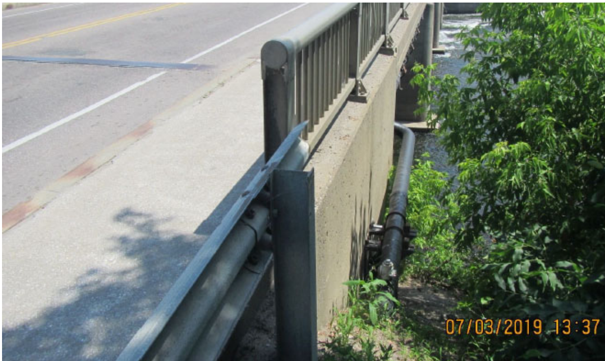
Figure 2. Facing south at northern end of bridge. Note utility alongside bridge and under abutment.
