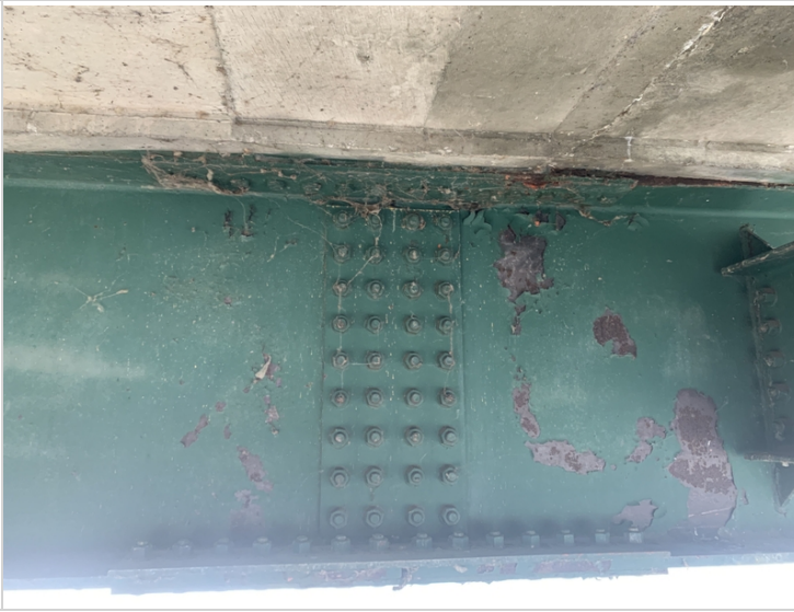
Beam 4 splice plate span 2
