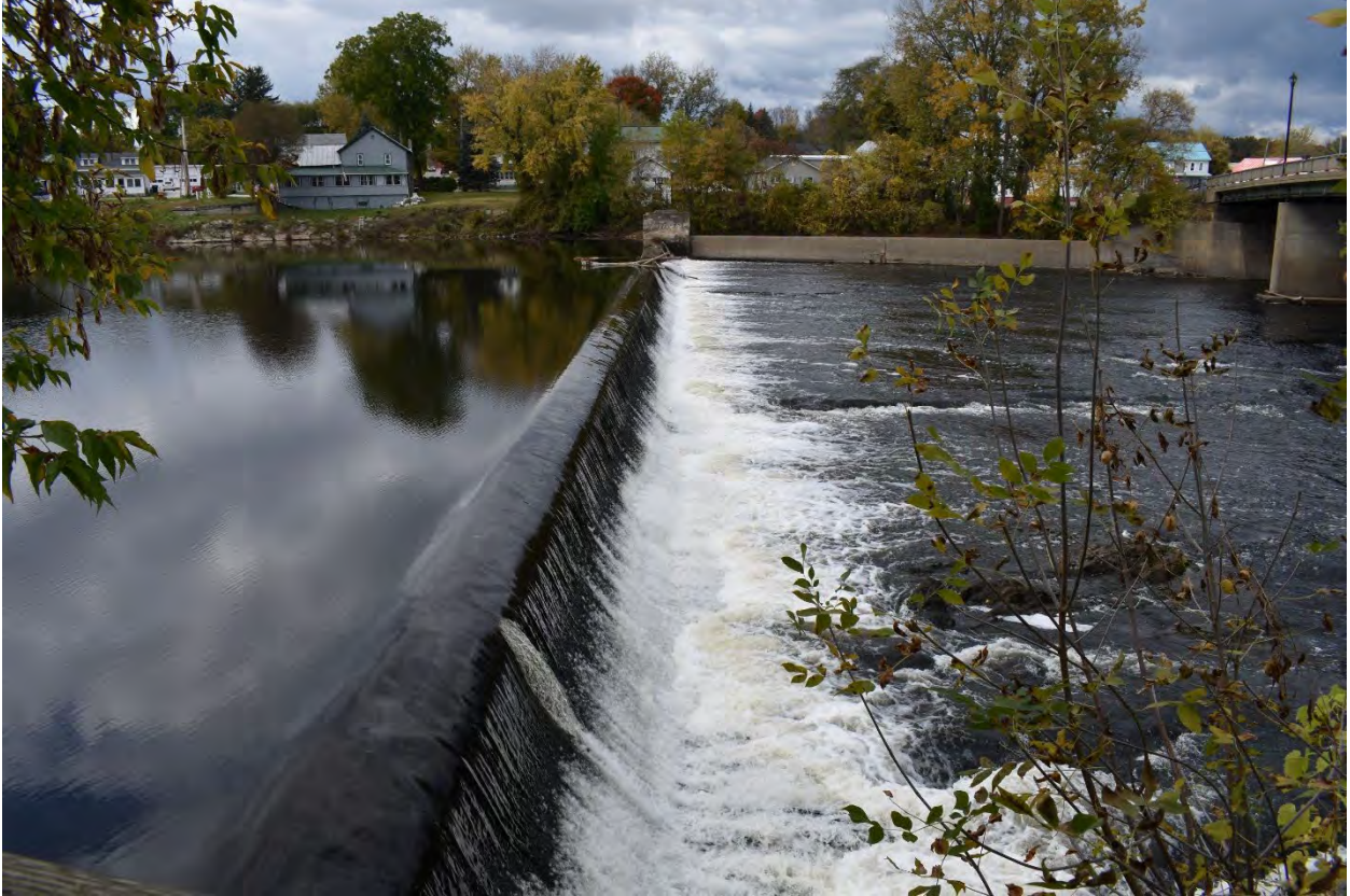
Figure 20. View northwest from the southwest quadrant of the proposed Swanton BF 036-1(16) Project in Swanton, Franklin County, Vermont. The photo was taken from the scenic overlook of the Swanton Dam adjacent to ASA 1. Note the bridge on the right of the photo.
