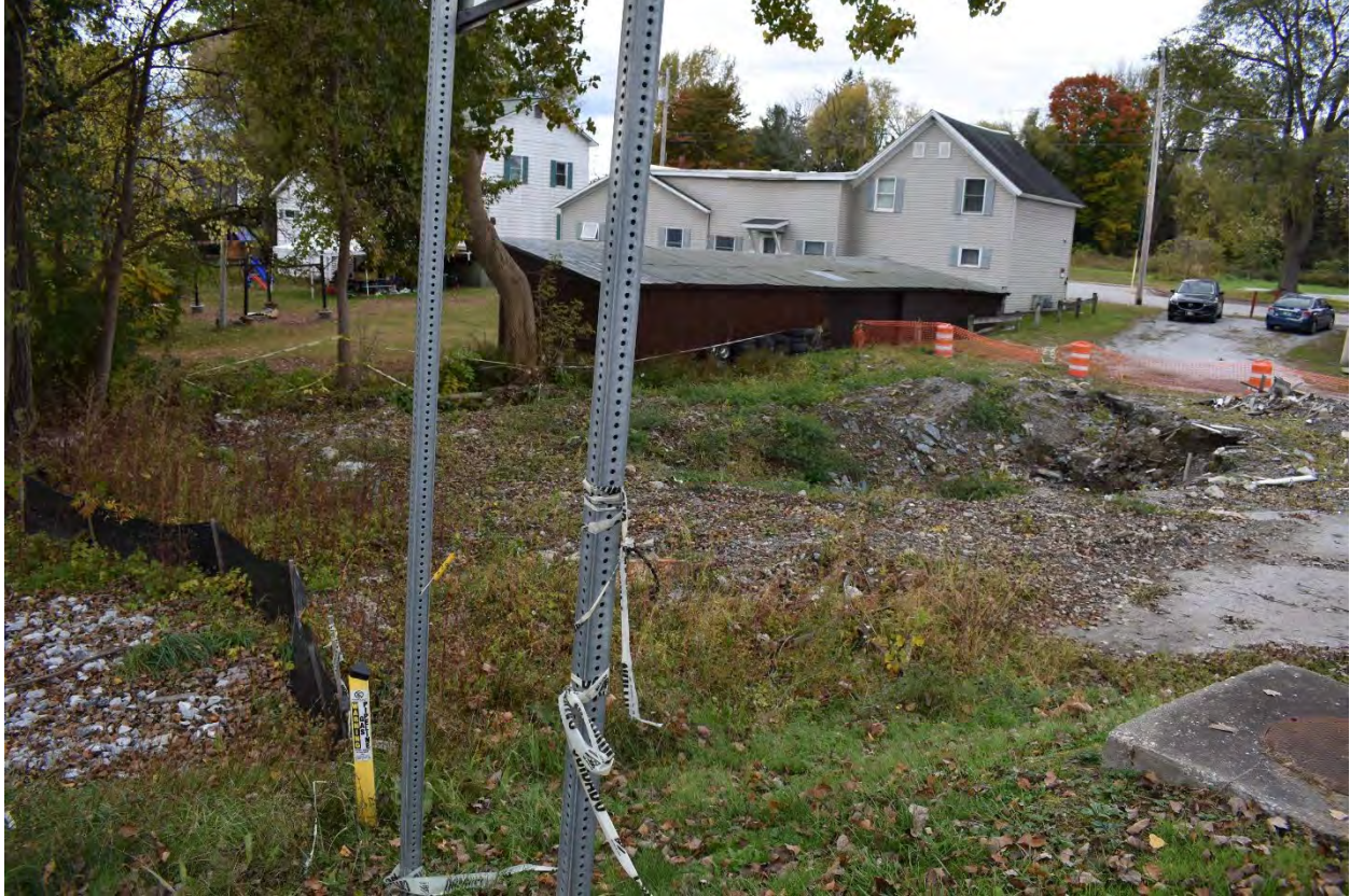
Figure 23. View southwest of the northwest quadrant of the APE of the proposed Swanton BF 036-1(16) Project in Swanton, Franklin County, Vermont, showing the foundation hole left from the removal of a building. ASA 5 includes the lawn visible in the background. The bridge is behind the photographer.
