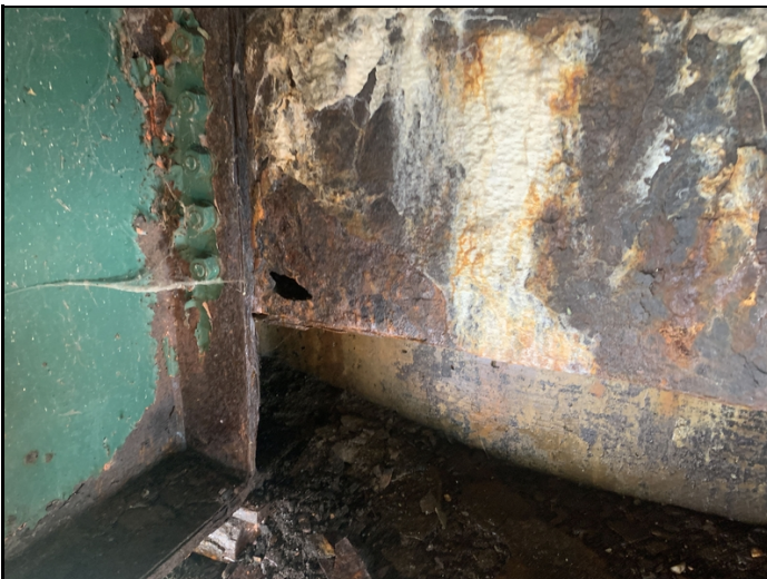
hole in the diaphragm
