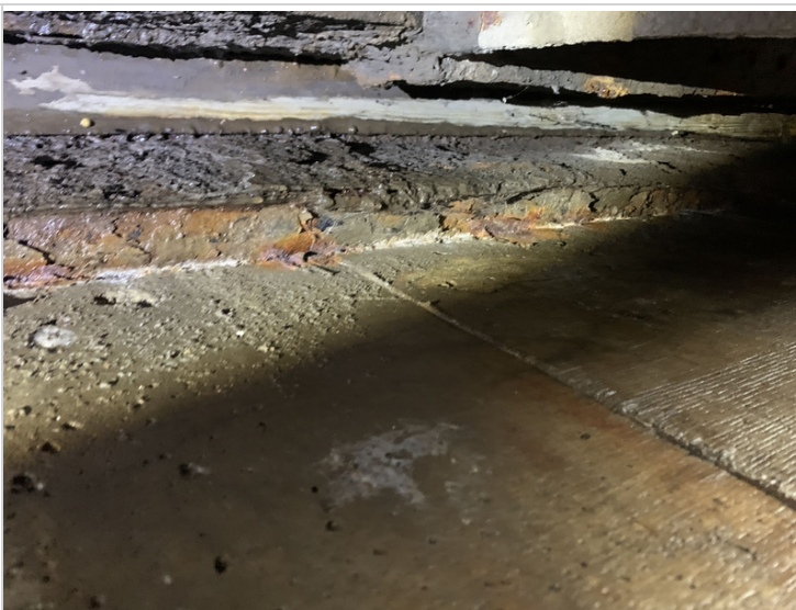
Abutment 1 joint
