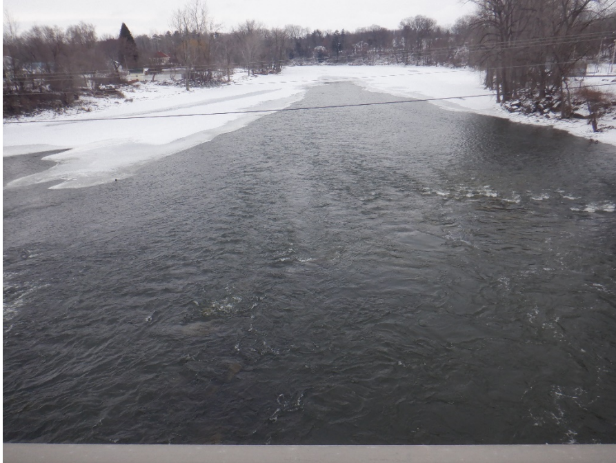
Photo 9: Bridge 8 - Looking Downstream (North)
