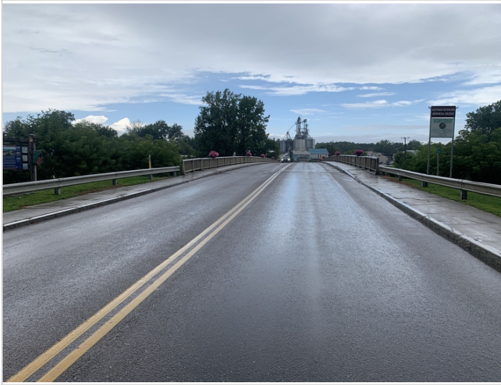
Approach looking west
