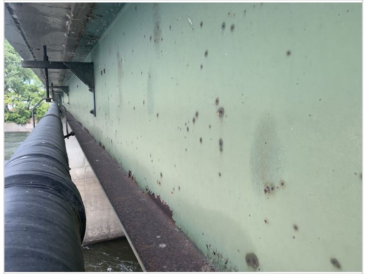
Beam 6 looking west
