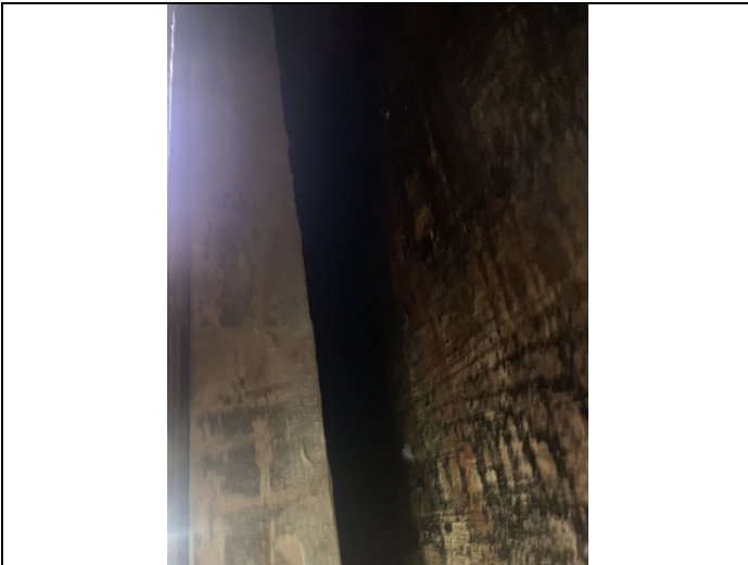
plywood temporary form work abutment 1
