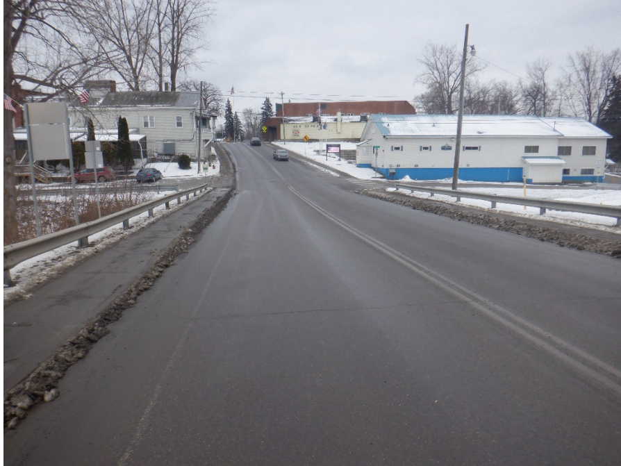
Photo 5: Bridge 6 – East Approach from Bridge, Looking East
