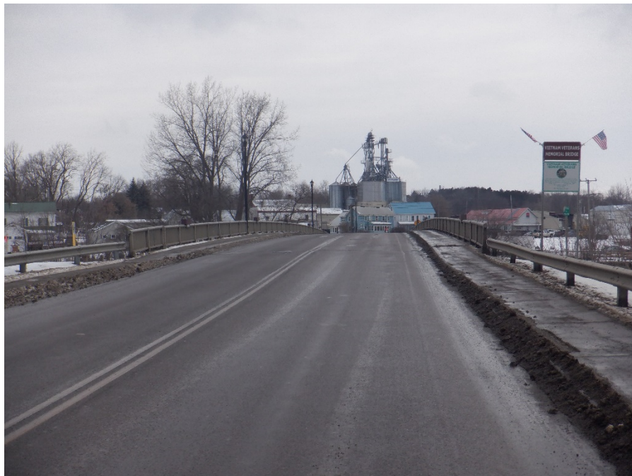
Photo 4: Bridge 6 – Bridge from East Approach, Looking West
