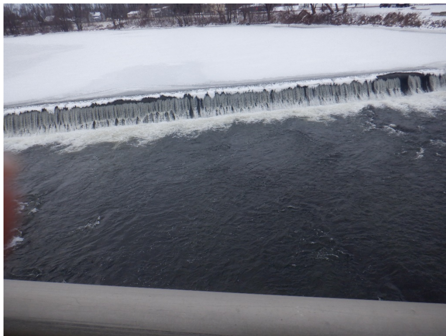
Photo 8: Bridge 6 – Looking Upstream (South)
