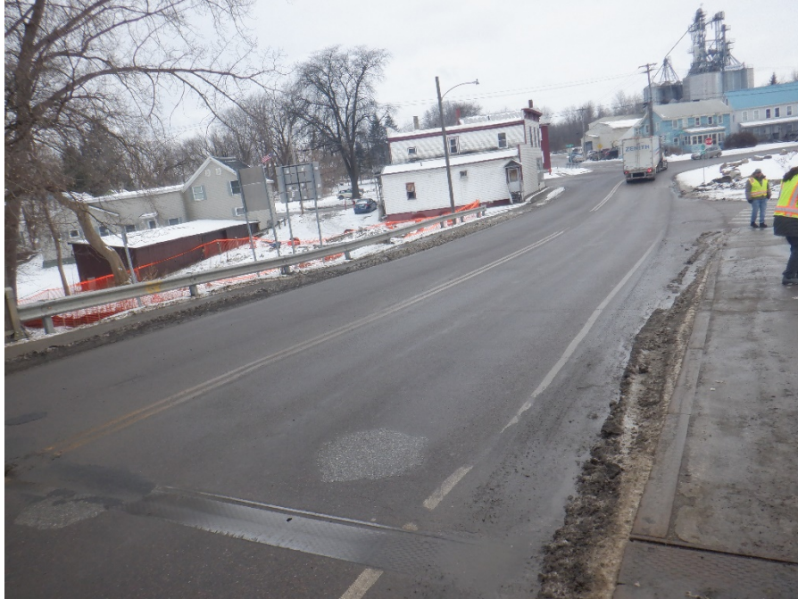
Photo 3: Bridge 6 – West Approach from Bridge, Looking West
